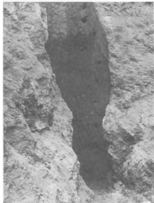
Figure 6 Roman Shafts Exposed in Early operations of RTC Above: Timbered shaft approximately 86 cm square. Below: Round shaft with hand/foot holes
